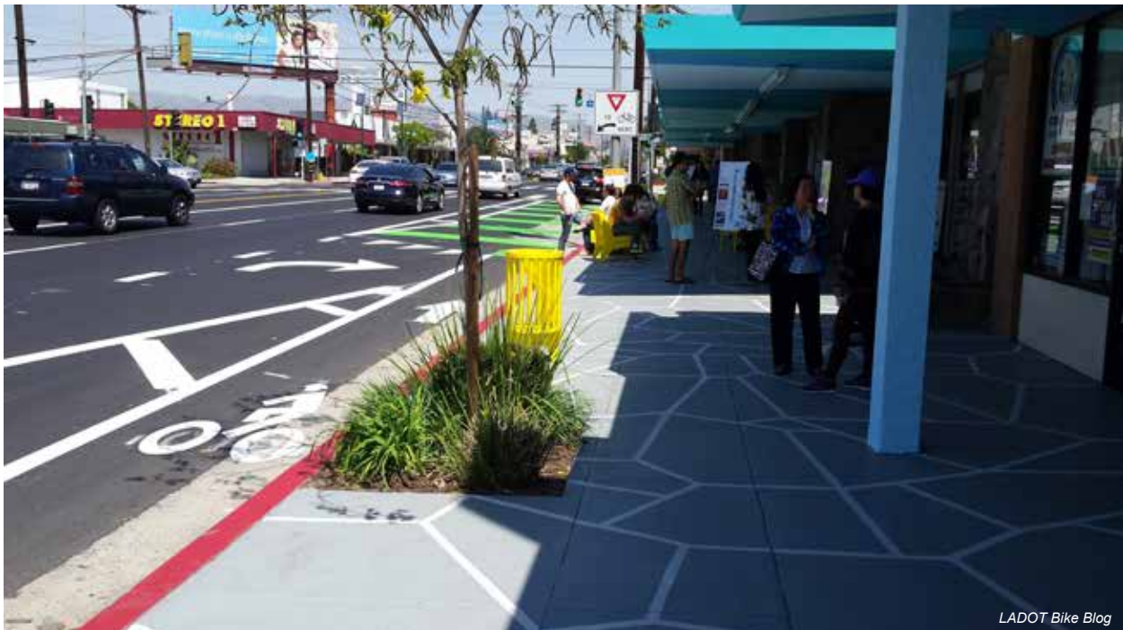
Reseda Boulevard, LA's first iteration of the Great Streets program shows how streets can facilitate low-stress travel with a parking protected bike lane and an attractive walking environment.
